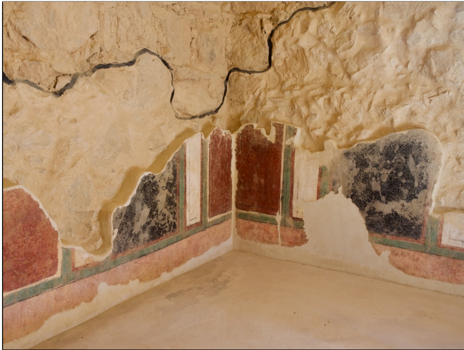
Inside of commander's house with painted plaster still covering the walls. Note the black restoration line (June 2022)
